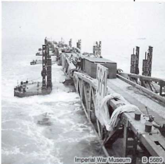
Figure 1. Sections of 'Whale' bridge. Image courtesy of RE Museum and IWM
