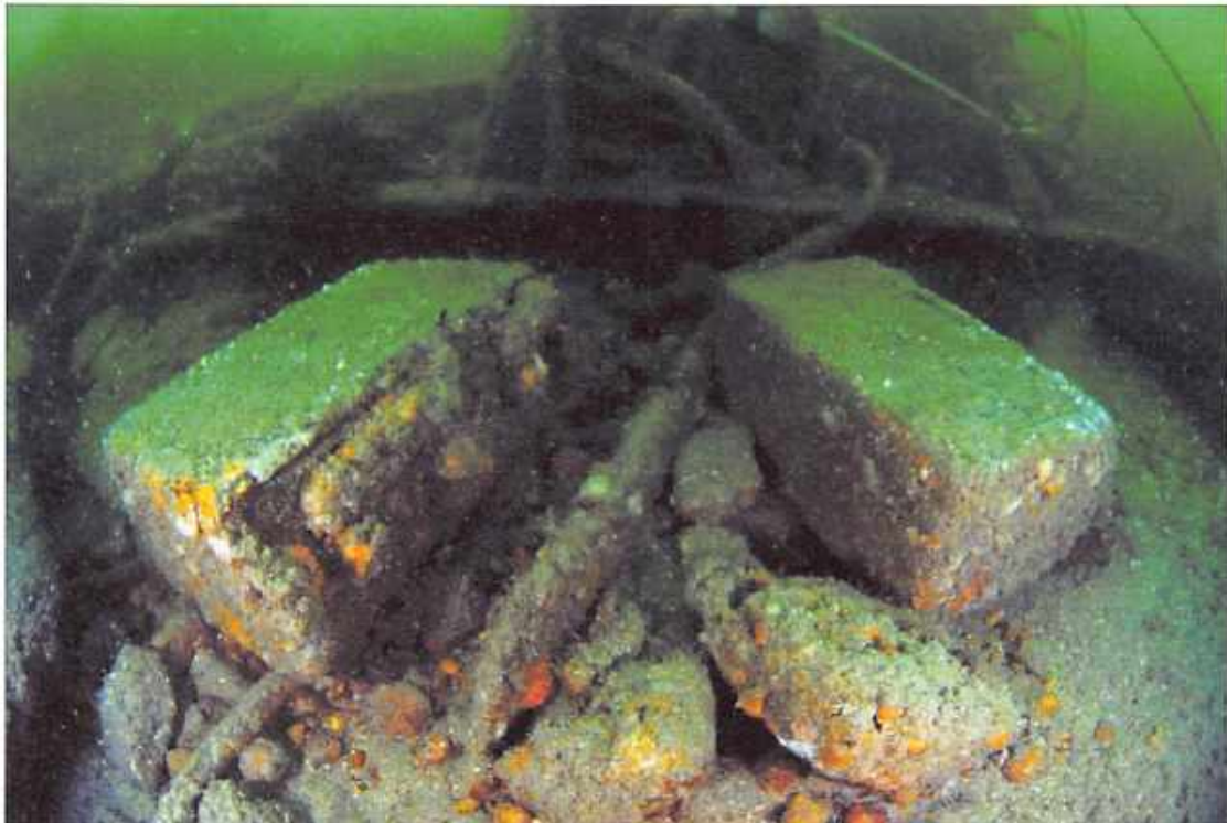
Figure 10 - Batteries and wiring (Image Martin Davies)
