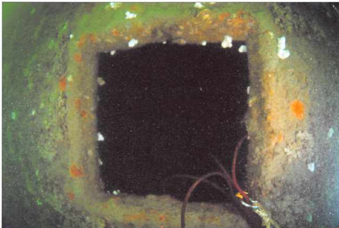
Figure 37 - Small opening / hole (Image Martin Davies)
