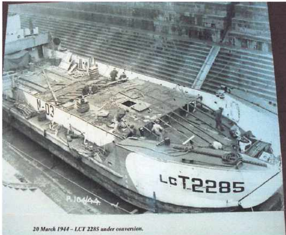
Figure 5 - LCT 2285 under conversion to fit tank ramps
