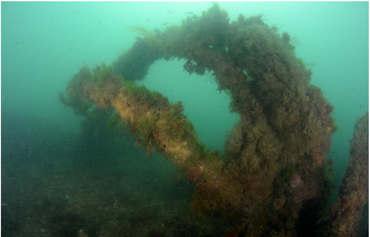
Figure 10 More of the steel re-bar has formed curved arches.
