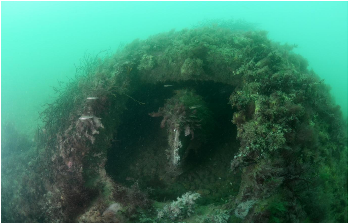
Figure 51 A nozzle in the opening of the dome.
