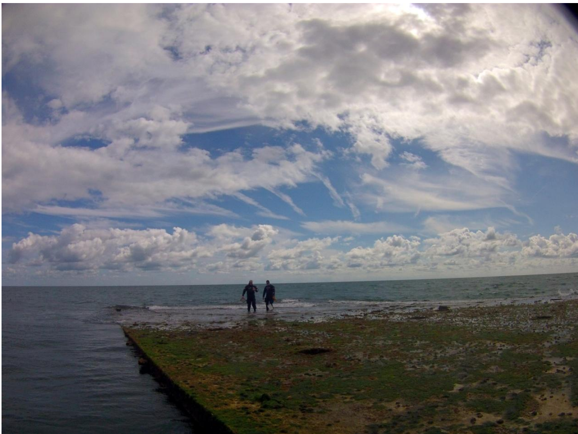
Figure 29 The Inner Mulberry is still very intact. Take care when walking on the top as there are holes appearing.
