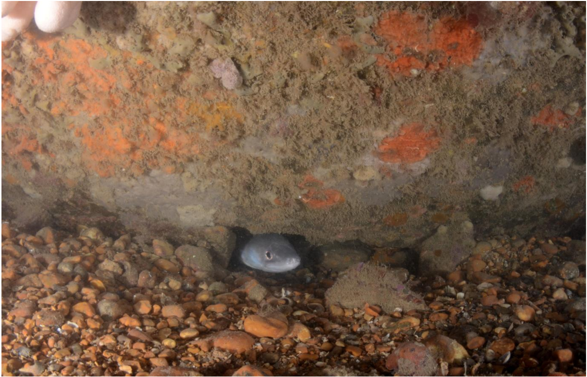
Figure 12 The base of the wall - a conger's home.
