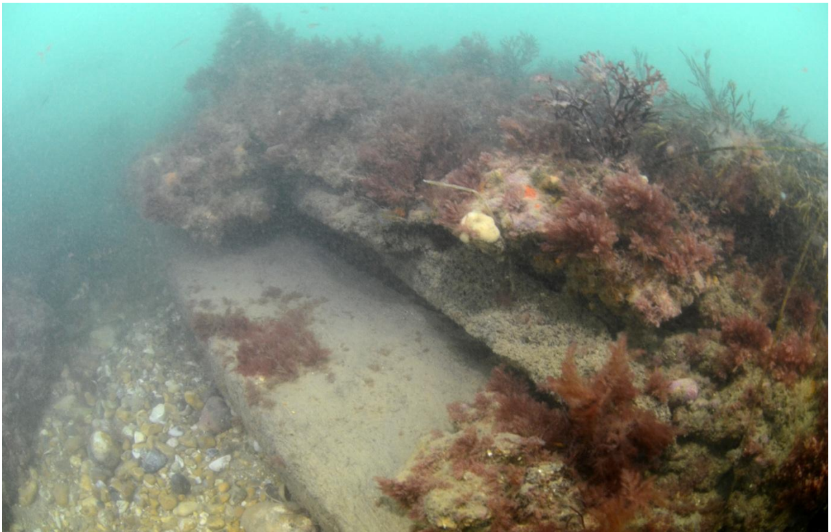
Figure 77 Layers of collapsed concrete.
