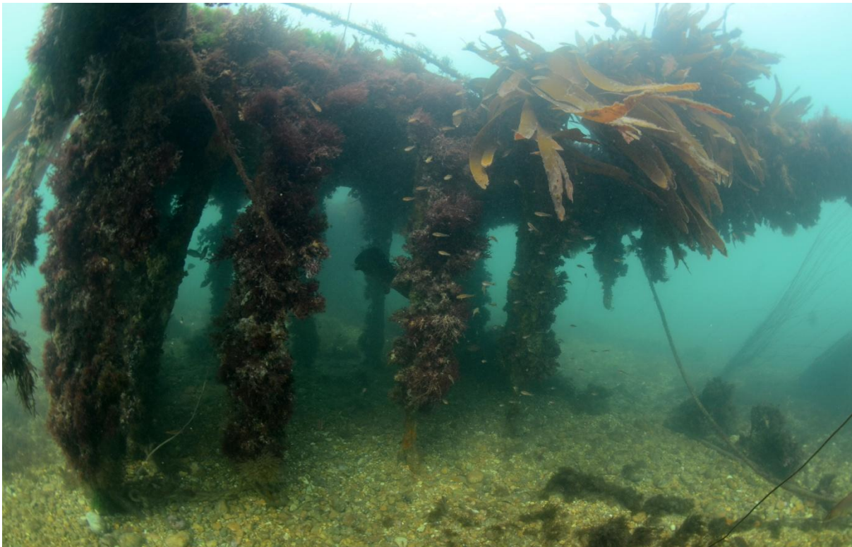
Figure 54 The end of the bridge pontoon has two extended arms.
