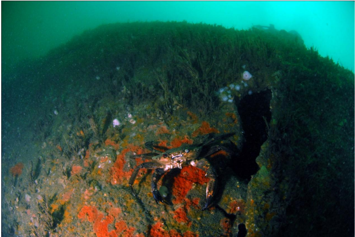
Figure 70 - the crack near the larger opening and velvet swimming crab.
