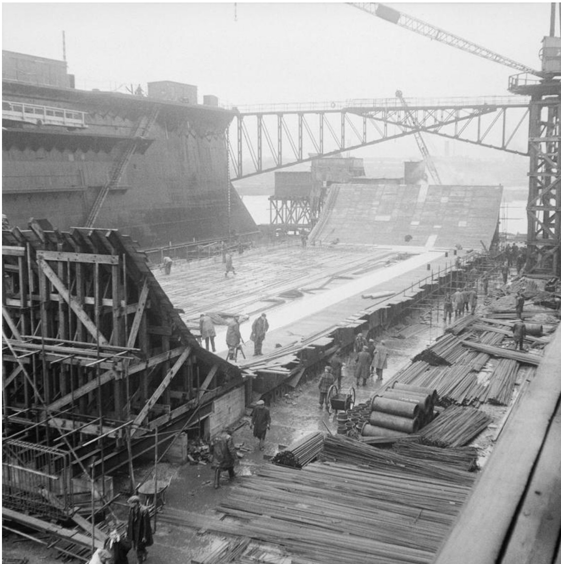
Figure 79 A concrete caisson or Phoenix, part of the Mulberry harbour for D-Day under construction 27 Jan 1944. IWM (H5379)
