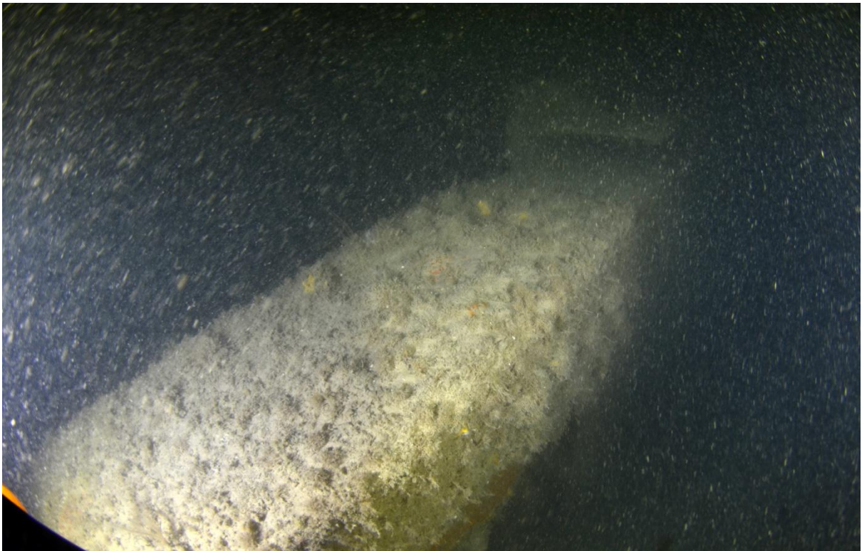
Figure 32 The top of one of the whale bridges showing the raised bolts/rivets typical of a whale bridge construction.
