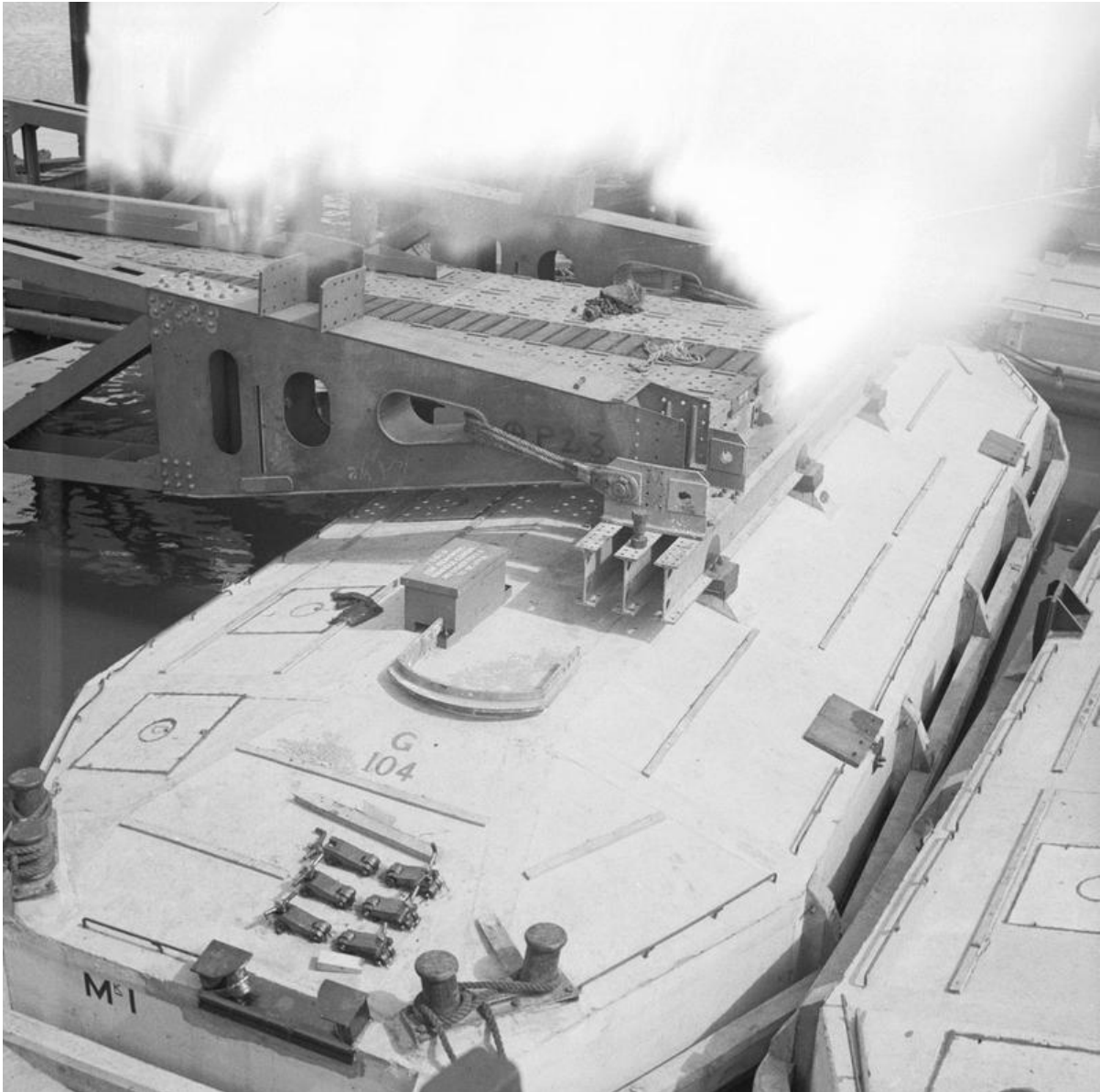
Figure 86 A section of the causeway being attached to a reinforced concrete float or Beetle. (IWM H39106).
