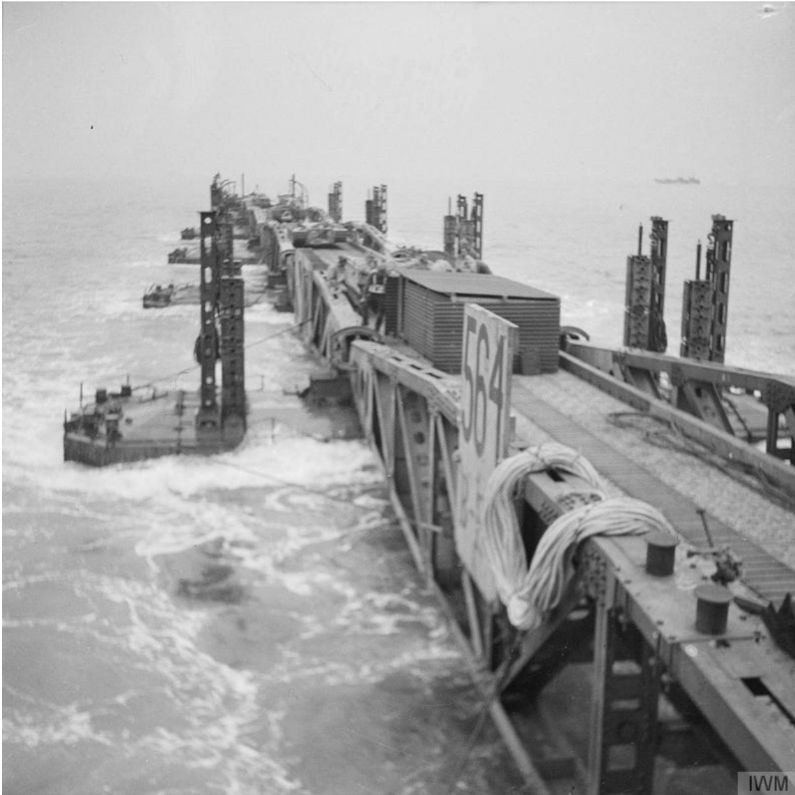
Figure 85 Part of the floating roadway being towed across the Channel to Arromanches. IWM (B5689)
