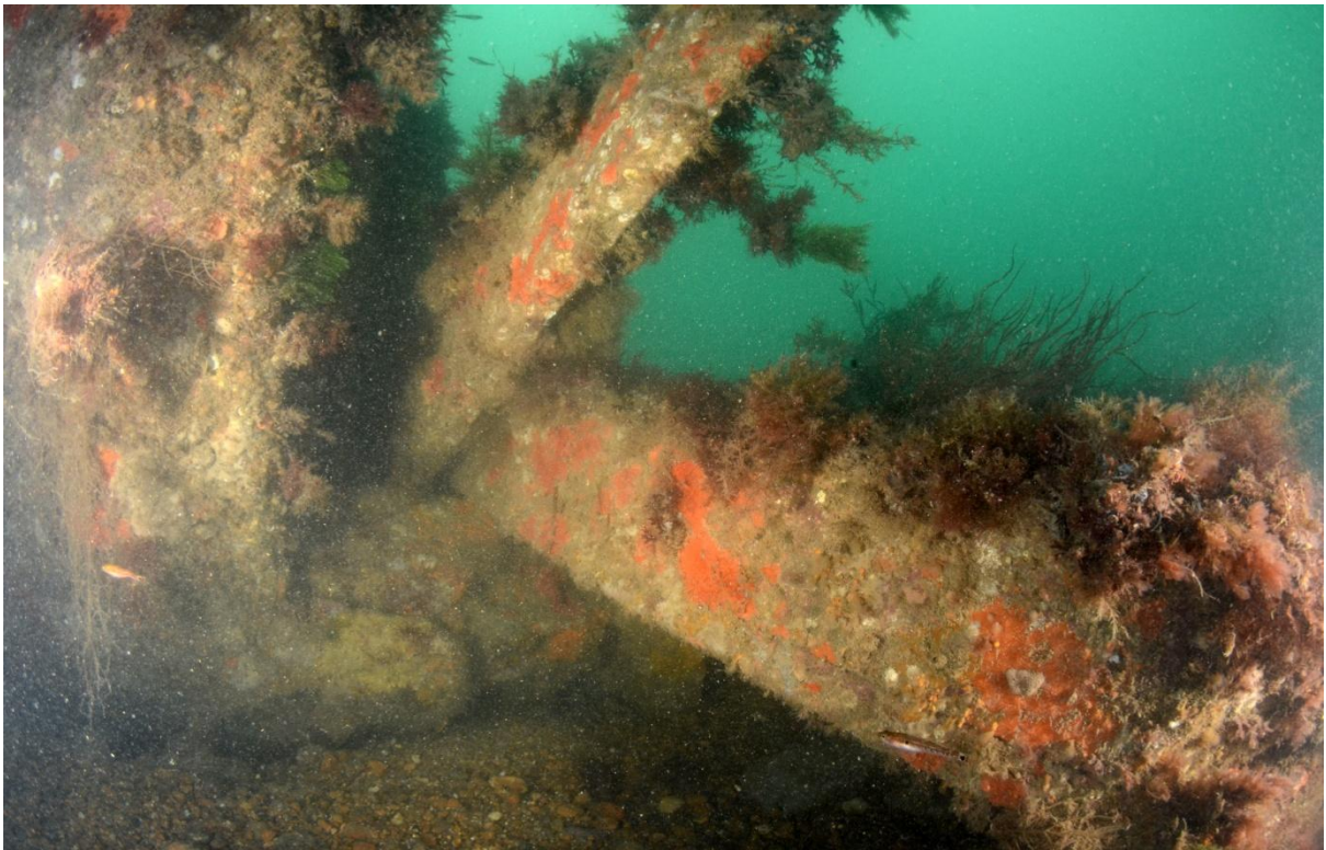
Figure 13 Large concrete girders have collapsed.
