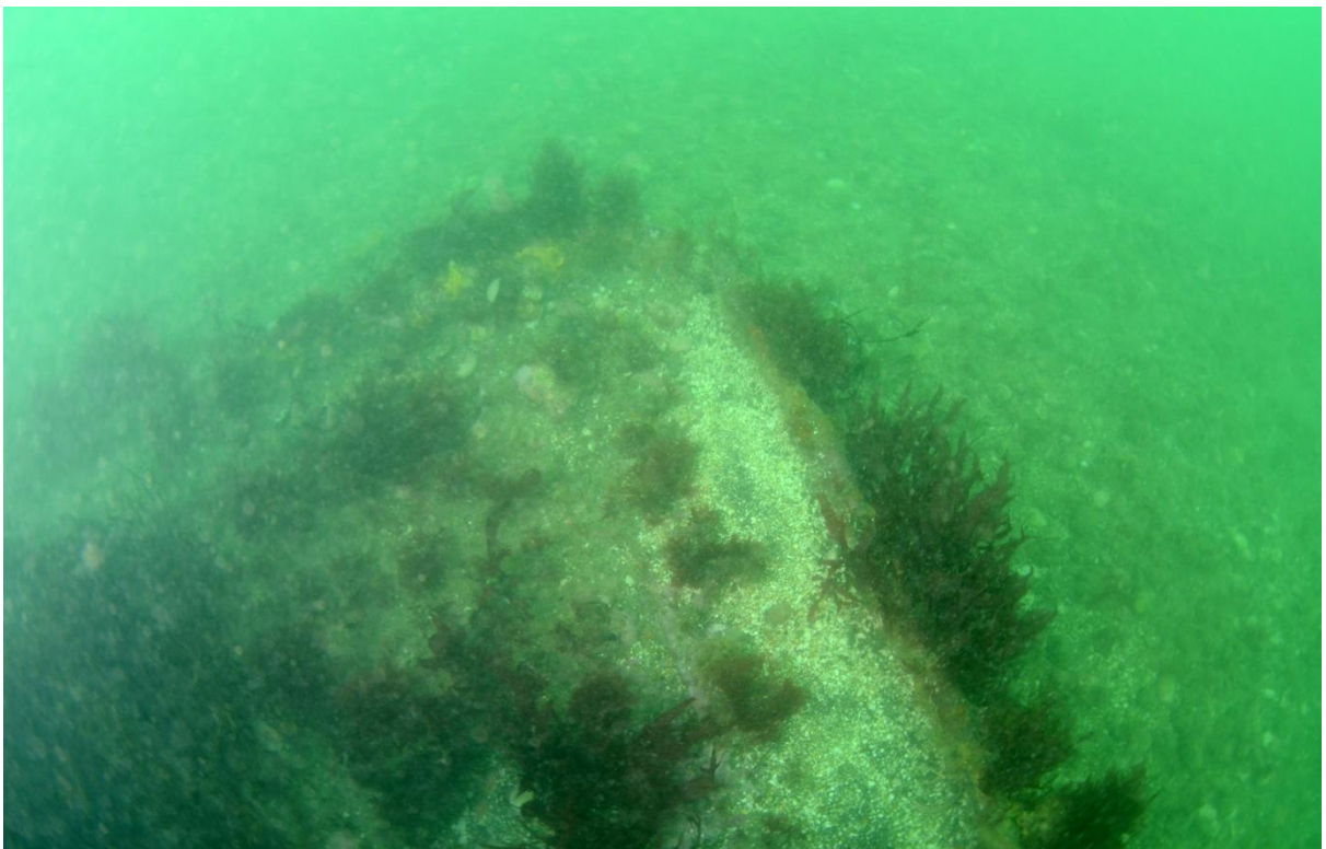
Figure 40 A view of the top of the pontoon structure.
