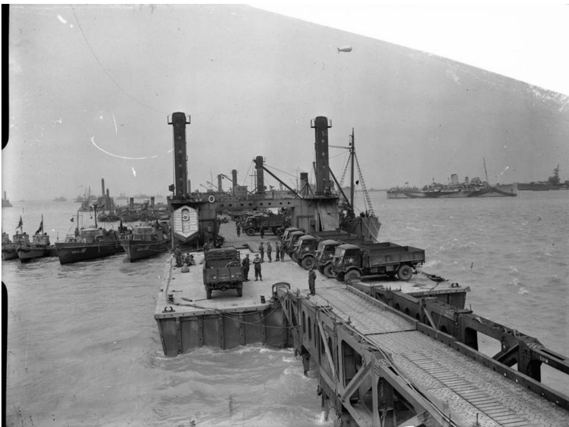
Figure 88 Buffer pontoon links a Spud Pier Head to a Whale bridge© IWM (A 24371)
