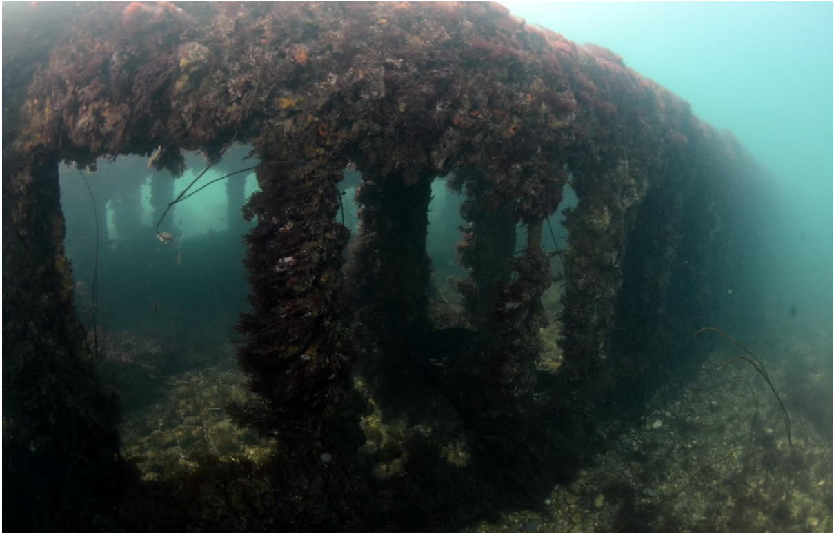
Figure 55 The pontoon stretches far into the distance - even with good visibility!
