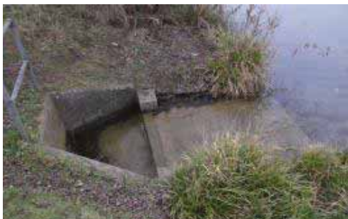
Photo 3 – Water overflow point for Balderton lake
