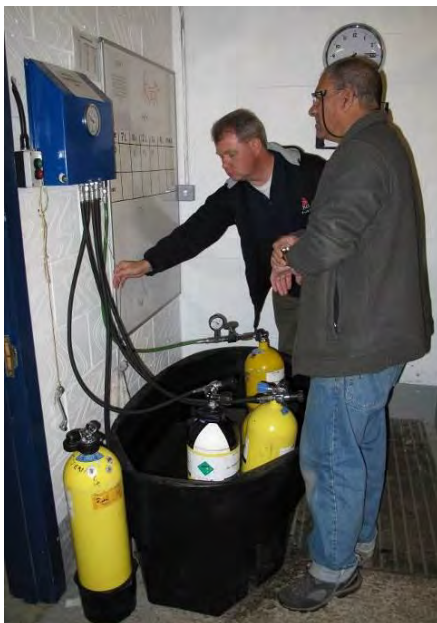
Our Compressor & Nitrox Facility
